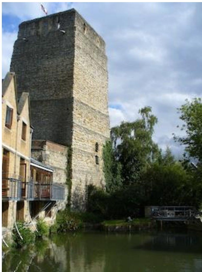
Castle Mill Stream and St George's Tower from Quaking Bridge
