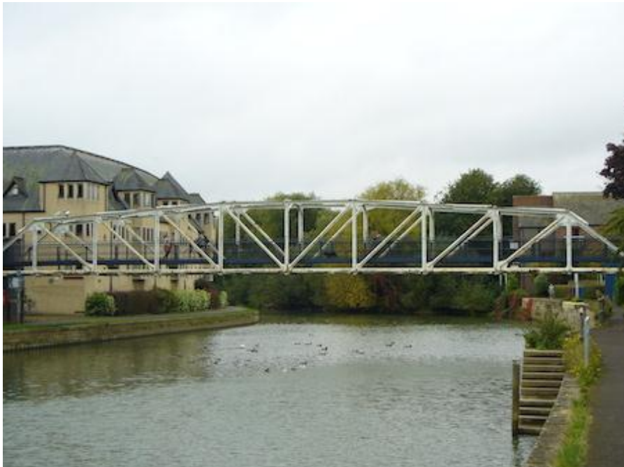
The former gasworks pipe bridge, now provides a footbridge linking St Ebbe's, to Grandpont to the south
