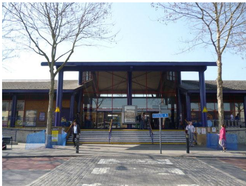
Oxford Station building completed in 1990 (© Robin Stones reproduced under Creative Commons License)
