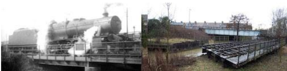
Top: The LMS Station as rebuilt at the Buckinghamshire Railway Centre Left: LMS Locomotive 8106 reversing over the fixed span 4 May 1942: RHG Simpson; Right: The LMS Swing Bridge today
