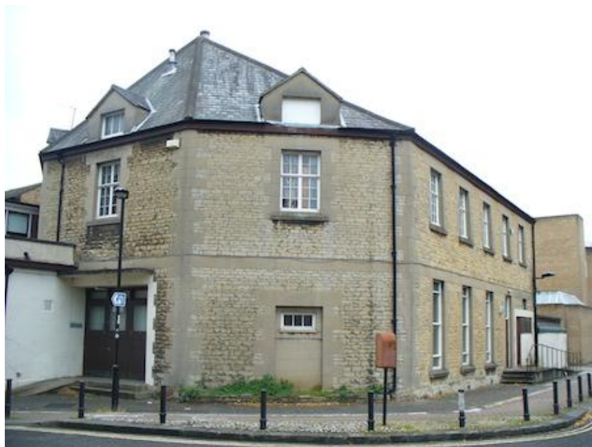
The former Baptist Chapel at No. 10a Littlegate Street was built in 1832, which continued in use until 1938
